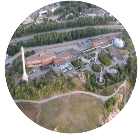
Viikinmäki wastewater treatment plant
